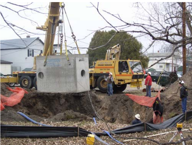
Installation of one of the Vortechnic oil-grit separators (2006).
