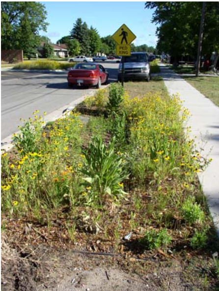
Rain garden #35 after enhancement with plugs and mulch (2007).
