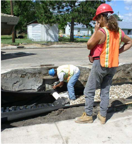
Rain garden #35 during construction (2005). An underdrain was added to enhance infiltration.
