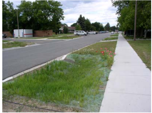
Rain garden #35 after planting (2006). Swale and prairie seed mixes were used, and plugs of native perennials were added.
