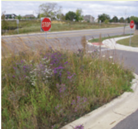
Bio-swales along Lake Street filter pollutants out of stormwater before the water reaches White Lake. (Prein & Newhof photo)
