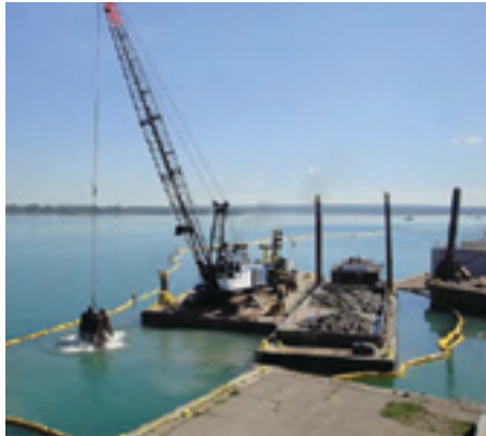
A clamshell dredge removes contaminated sediment from the lower Sheboygan River. (U.S. EPA photo)
