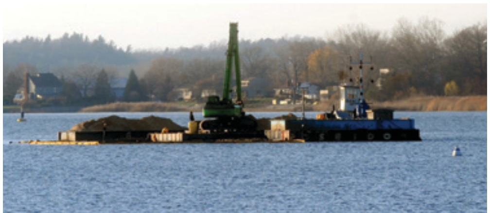
A dredge removes contaminated sediment from the bottom of Muskegon Lake. (U.S. Environmental Protection Agency photo)
