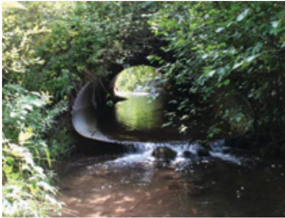
This culvert in Troutmere Creek was above the average water level, which prevented fish passage. (U.S. Fish and Wildlife Service photos)
