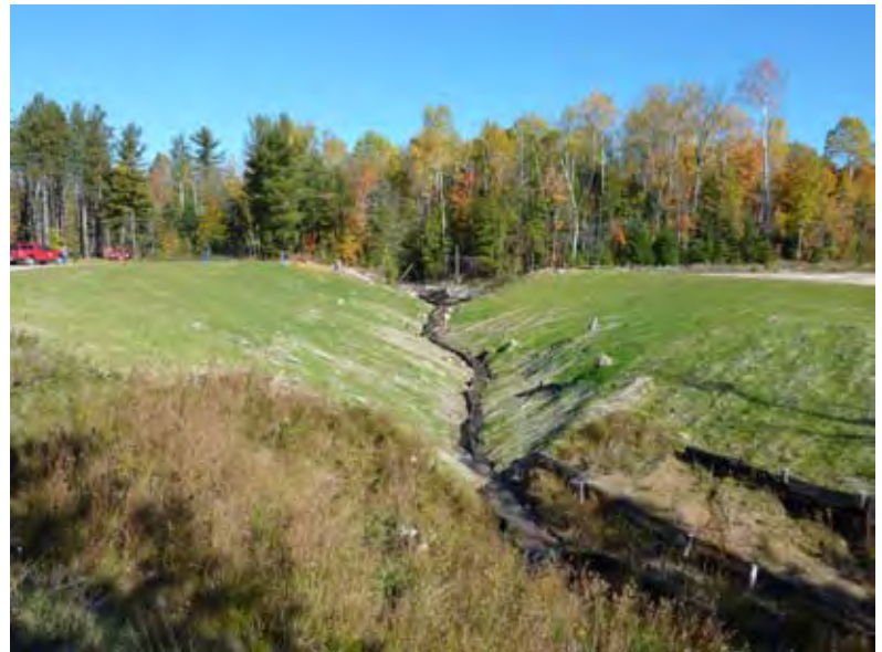
At this site, the barrier was completely removed and no grade control was installed: the stream was allowed to cut through sediment to establish a new channel and floodplain.
