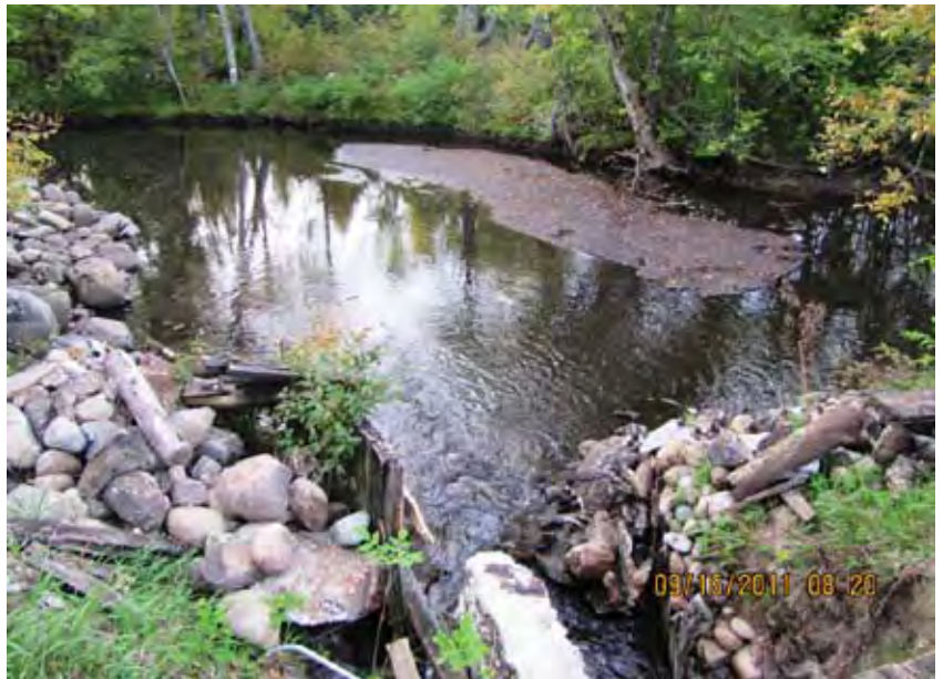
It is important to plan management of sediment movement, including accumulation of sediment downstream as shown above. Photo courtesy of the USFWS.
