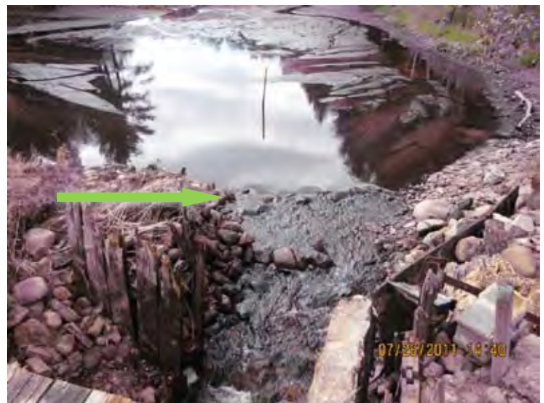
The small cross vane in the upper photo was removed, which allowed the second cross vane in the lower photo to control water elevation. Photo courtesy of USFWS.
