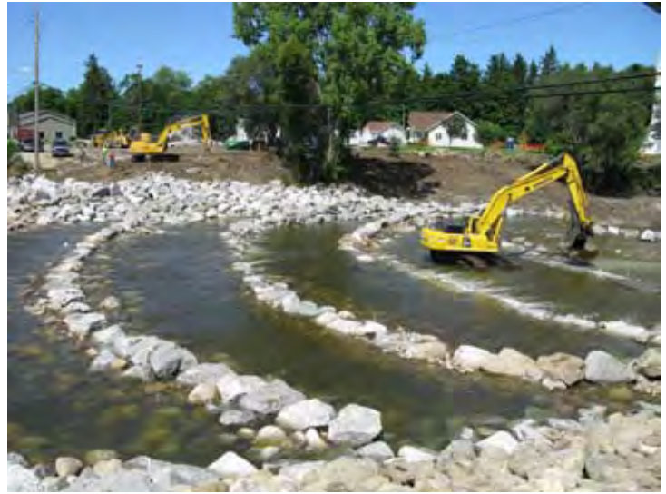
In this situation, grade control structures were used to maintain water levels while allowing fish passage. Photo courtesy of USFWS.
