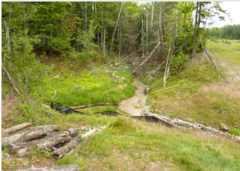
Above, Myers Creek impoundment before dam removal. Below, the establishment of the new channel through the former impoundment after the removal.
