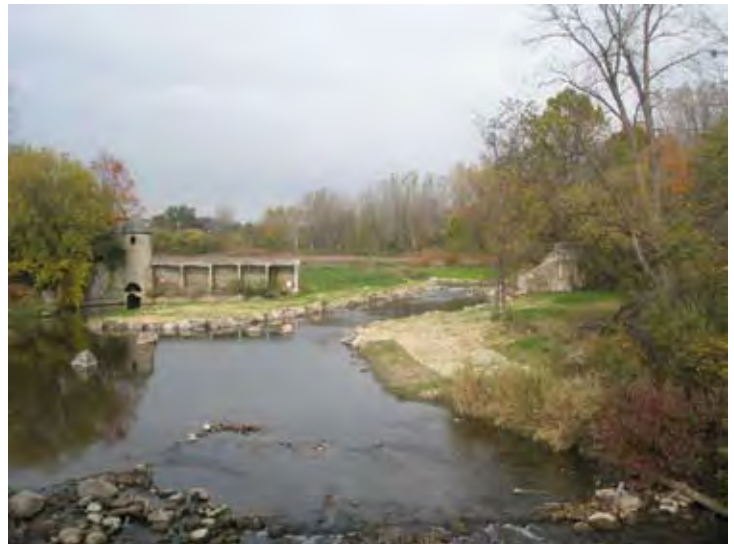
This dam was partially removed, allowing for fish passage while protecting a historical structure. Photo courtesy of Jim Francis, MDNR.
