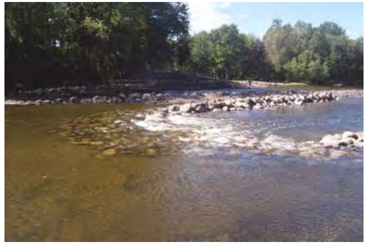
Here, the dam was completely removed and a grade control structure was installed. Photo courtesy of Ralph Reznick, MDEQ.
