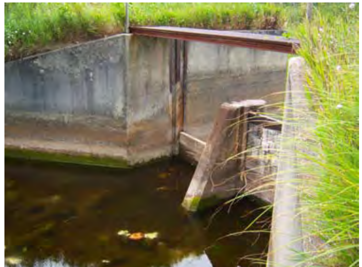
A typical small dam with stop logs to control water level.
