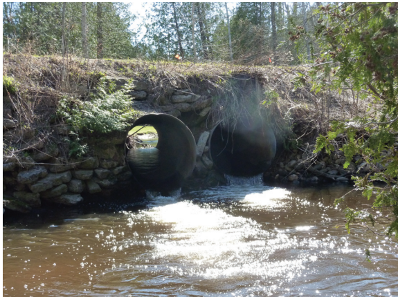
Photo 4-5: An old road crossing of a river that prevented fish passage and allowed sediment to pollute the river.
